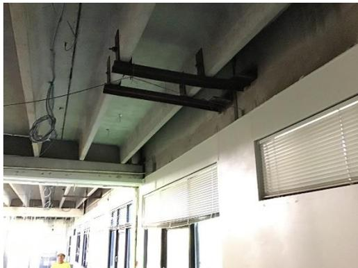
Structural Supports for Roof Openings
